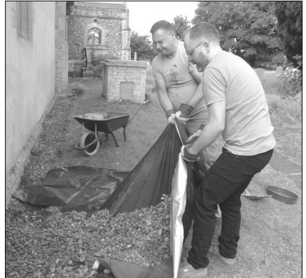
Clearing the churchyard and working on the French drain.
